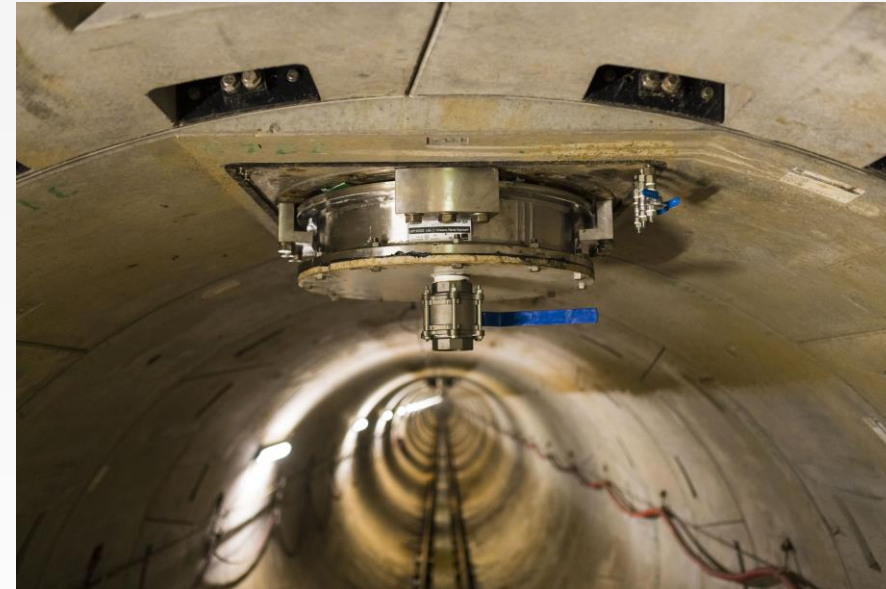
Step 3: Riser completion including temporary bulkheads, removed prior outfall tunnel flooding
