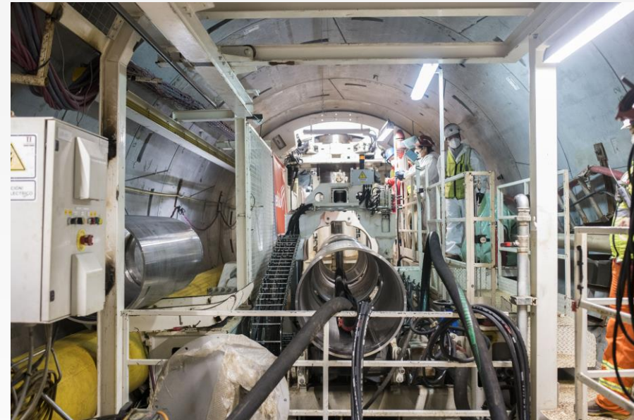
Step 2: Mechanized Riser Installation by jacking upward riser segments.
